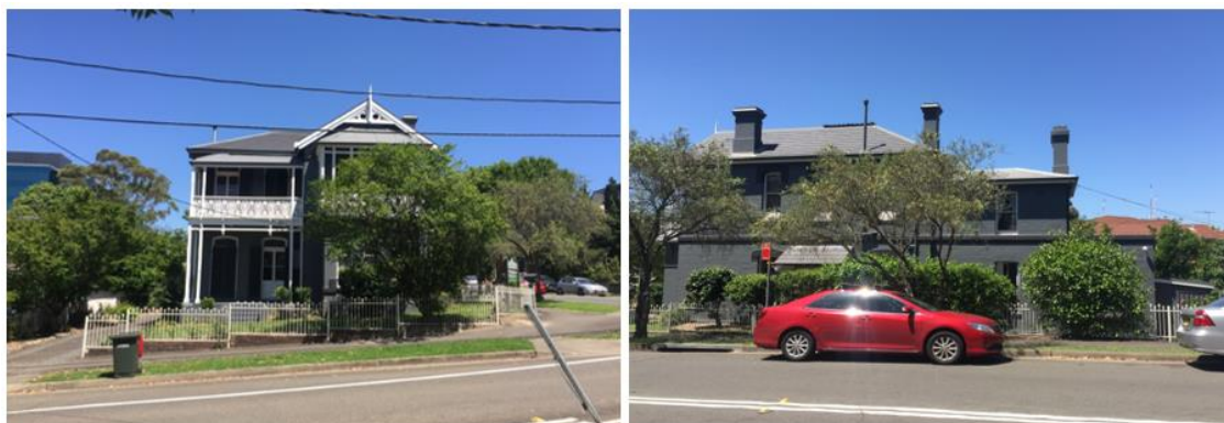
Figure 8 – View of 53 Sorrell St (left) and side view from Harold St, part of subject site and heritage item.
